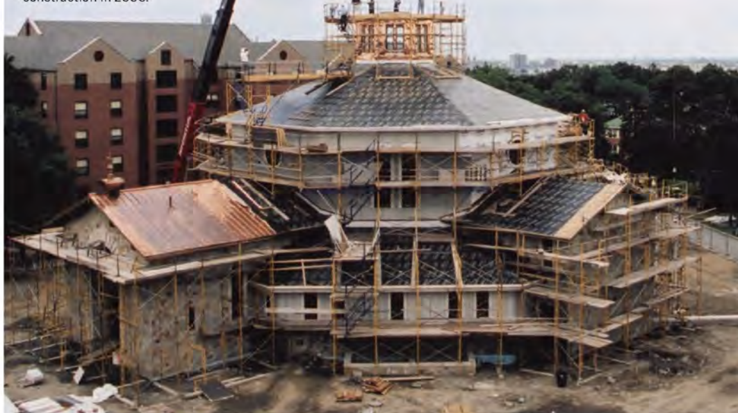
St. Dominic Chapel under construction in 2000.
